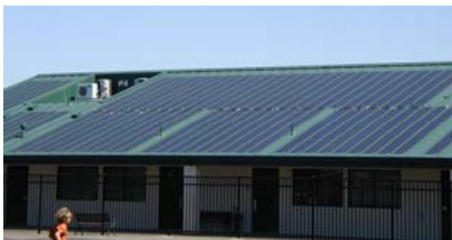
Greenbrook School, 130KW PV System
